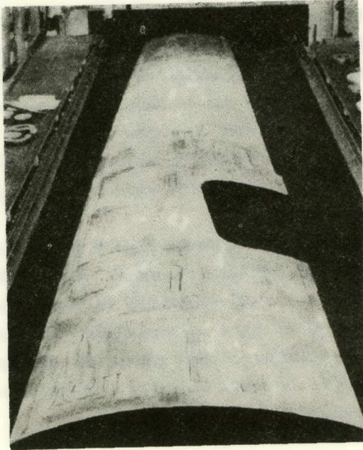
Fig. 4. A long wing panel after shot-peen forming.
